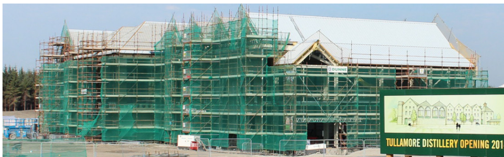
Tullamore DEW distillery under construction at Clonminch off the by-pass
