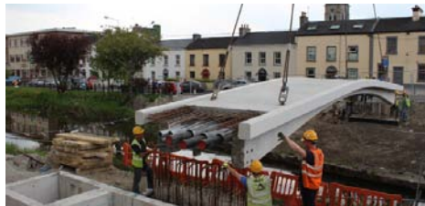
New pedestrian bridge being lowered into position alongside Kilbeggan Bridge
